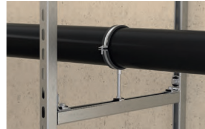
Pipe fixing on frame construction
